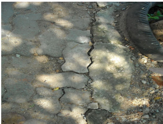
Fig. 6.15 Poor support from edge restrain
