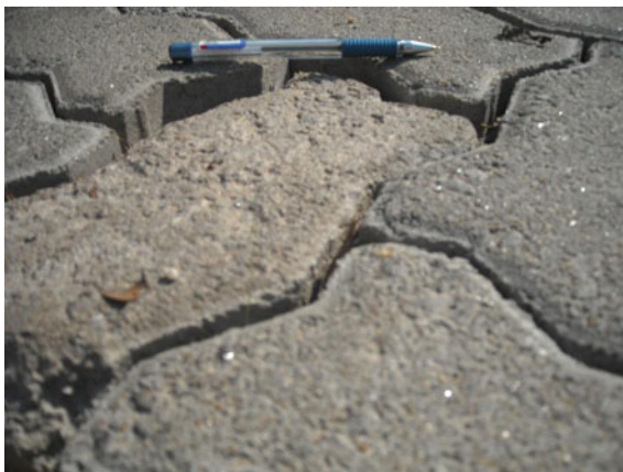
Fig. 6.3 Jointing material has been lost from pavers at leads resulting in loss of interlock
