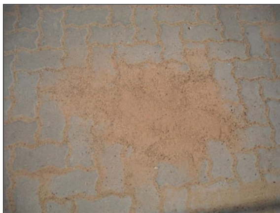
Fig. 6.6 Sand patches on CBP surface
