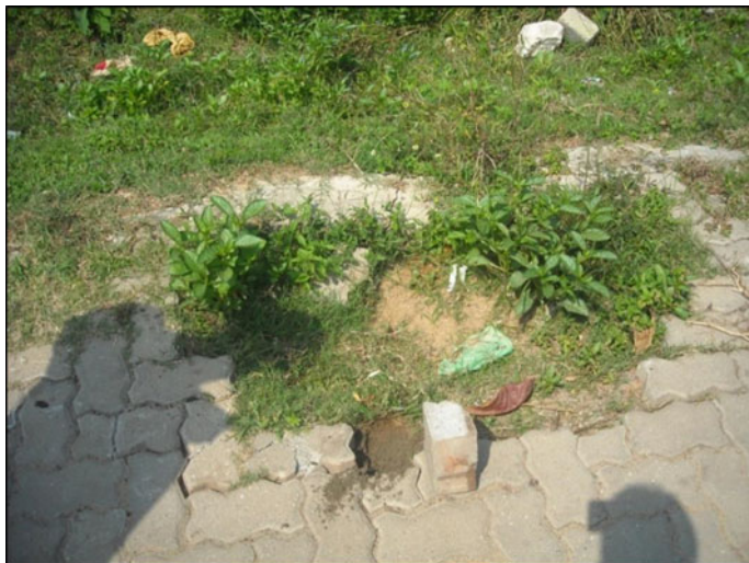
Fig. 6.13 Wider gap and failed blocks
