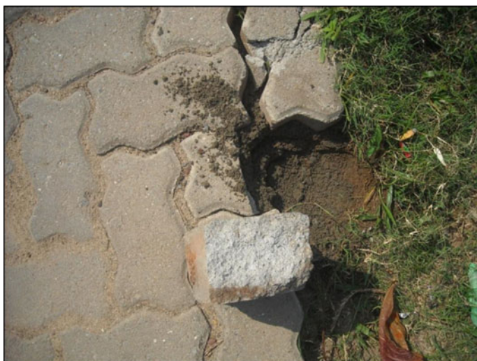
Fig. 6.14 Washout of the sand bed
