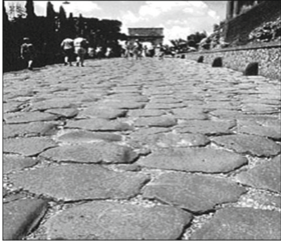
Fig. 1.1 The early interlocking pavement—Roman Appian way (ICPI, 2004)
