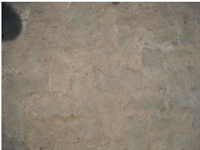
Fig. 6.18 CBP section with rigid joints (filled with cement mortar)
