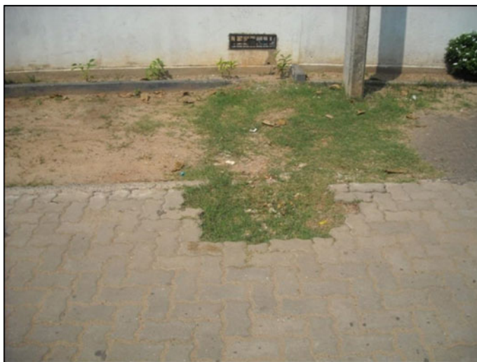
Fig. 6.12 No edge restrain in the section of the road
