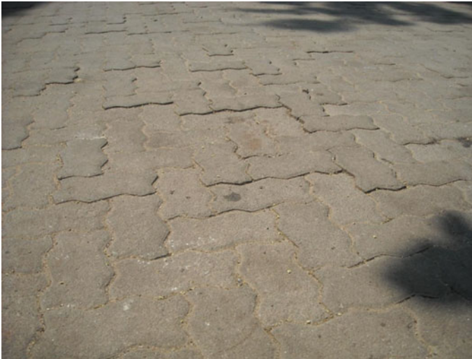
Fig. 6.17 Faulting of a CBP road
