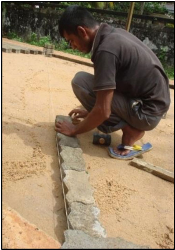
Fig. 5.8 Angle laying of the stretcher bond pattern
