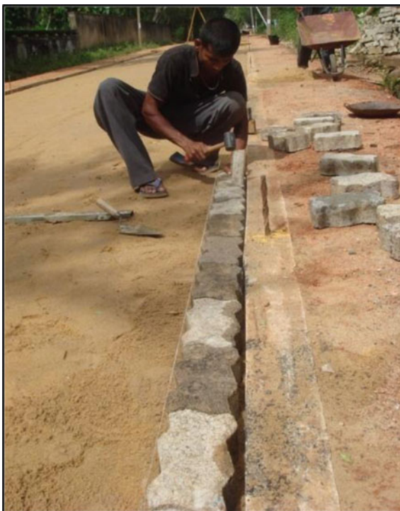
Fig. 5.10 Laying of stretcher bond pattern to 90^\circ or 0^\circ
