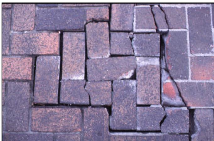
Fig. 6.19 Failure of rigidly set brick pavers at Bellevue Metro, Washington State, US ('John Knapton's Pictorial Guide to Paving through the Ages.', n.d.)
