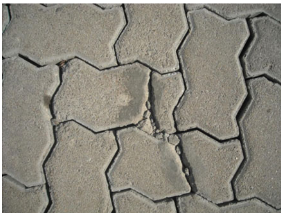
Fig. 6.4 Failure of surfacing on a car park deck as a result of jointing sand being washed/vibrated into bedding course
