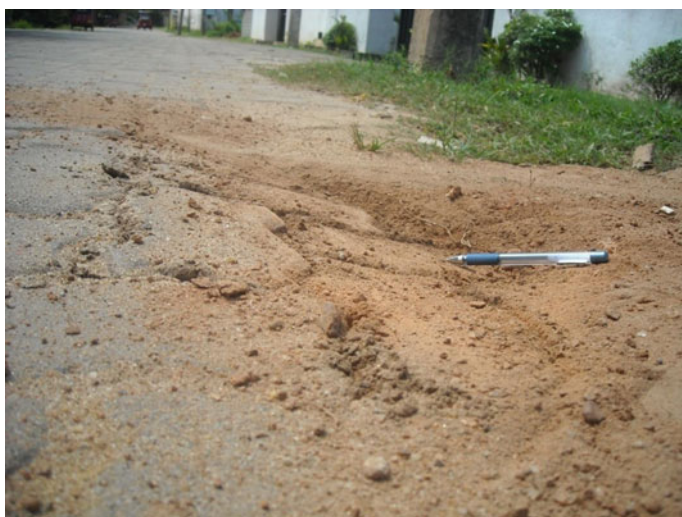
Fig. 6.16 Base failure
