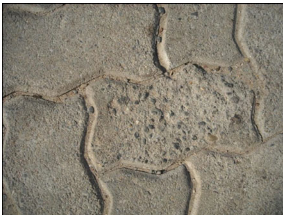
Fig. 6.8 Washout of blocks
