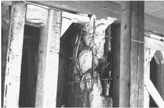
Figure 12.14 Timber propping of a damaged column; Kalamata, Greece (1986).
