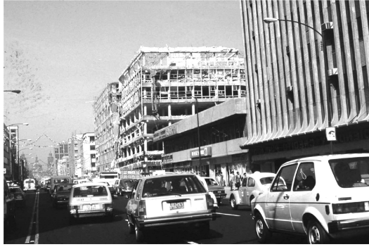
Figure 11.36 Large-scale damage at the upper floors of a flexible high building, Mexico City (1985).
