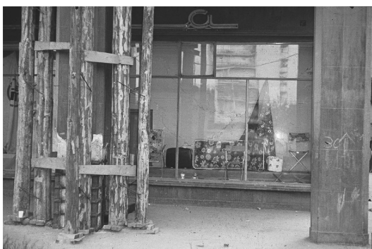
Figure 12.13 Timber propping of a damaged column; Bucharest, Romania (1977).
