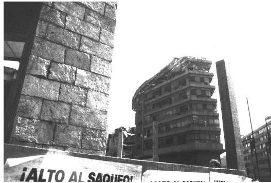
Figure 11.48 Consequences of soil liquefaction on a high building in Mexico City (1985).
