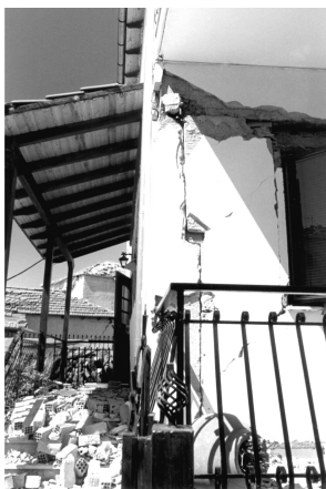
Figure 11.32 Damage to masonry walls: Kozani, Greece (1996).
