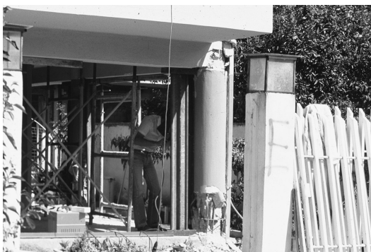
Figure 11.3 Column damage due to high axial compression and cyclic bending moment: Kalamata, Greece (1986).
