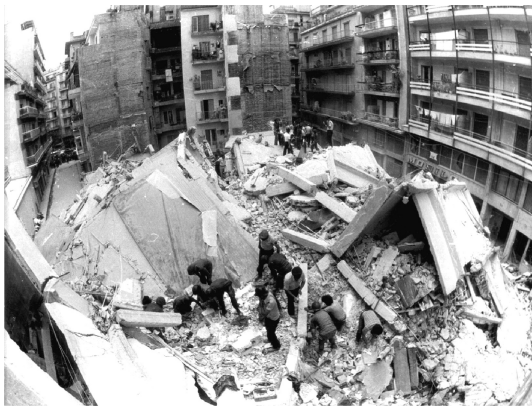
Figure 11.49 Collapse of an eight-storey corner building in Thessaloniki, Greece (1978).
