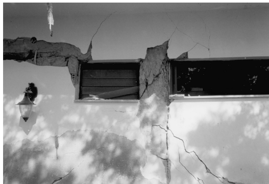
Figure 11.8 Explosive cleavage failure of a short column: Kozani, Greece (1996).
