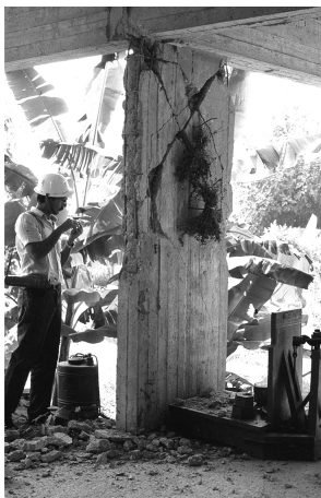
Figure 11.35 Column damage of the open ground storey (pilotis system), Kalamata, Greece (1986).
