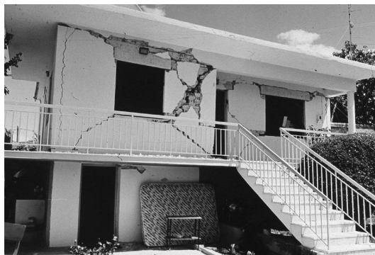
Figure 11.31 Damage to masonry walls: Kalamata, Greece (1986).
