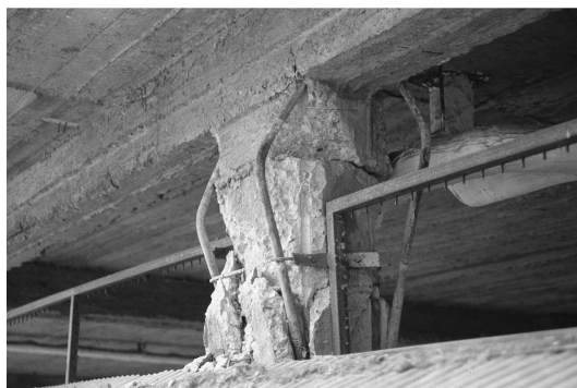
Figure 11.9 Explosive cleavage failure of a short column: Kalamata, Greece (1986).
