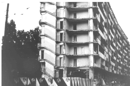
Figure 11.44 Collapse of a building with a flexible ground floor: Bucharest, Romania (1977).
