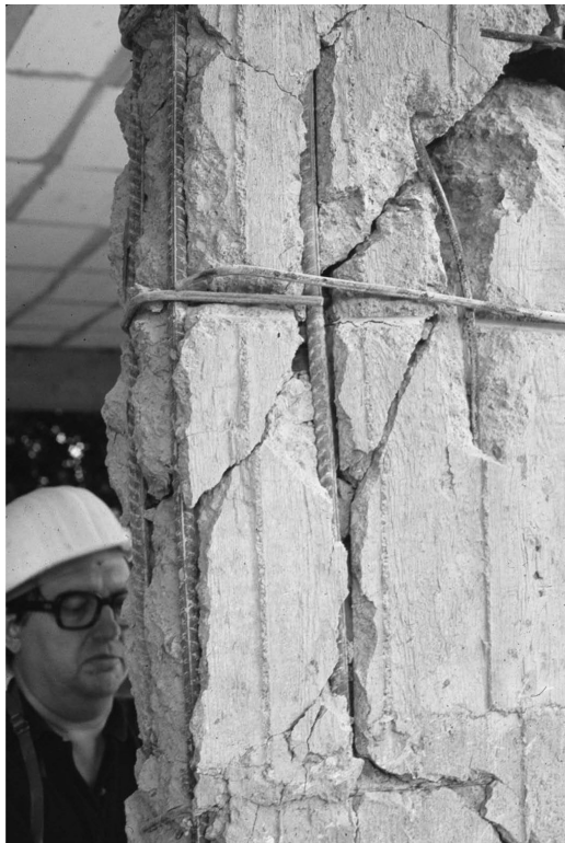
Figure 11.16 Shear wall failure due to shear: Kalamata, Greece (1986).
