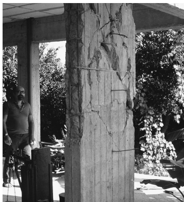
Figure 11.6 Column damage due to high axial compression and cyclic shear: Kalamata, Greece (1986).
