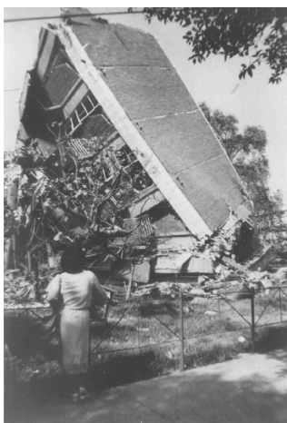
Figure 11.40 Torsional collapse of a building in Mexico City (1985).
