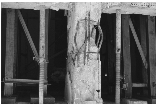
Figure 11.5 Column damage due to high axial compression and cyclic shear: Kalamata, Greece (1986).
