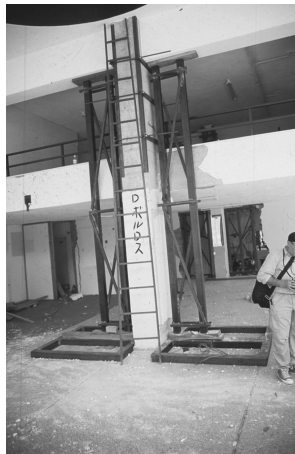
Figure 12.15 Steel profile props for the repair of a damaged column; Kalamata, Greece (1986).
