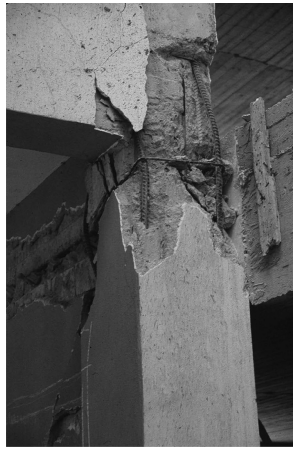
Figure 11.26 Failure of an exterior joint in a multi-storey building: Kalamata, Greece (1986).
