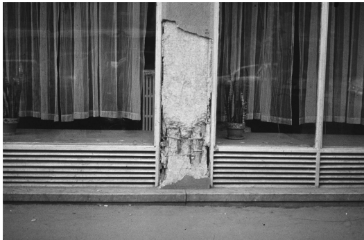
Figure 11.2 Column damage due to high axial compression and cyclic bending moment: Bucharest, Romania (1977).
