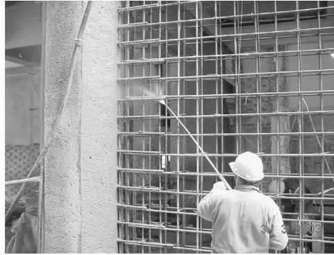
Figure 14.1 Dedusting and wetting of the old concrete and reinforcement at the complex of the Army Pension Organization (Athens).
