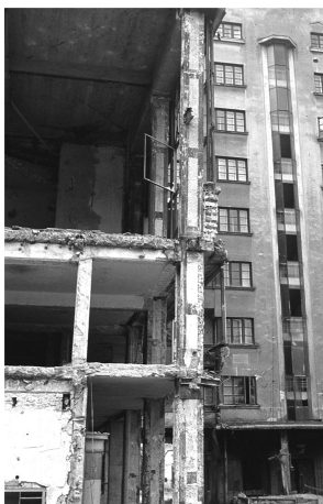
Figure 11.46 Collapse of a building in Bucharest during the 1977 earthquake. The building, as depicted in the illustration, had been repaired after the 1940 earthquake.
