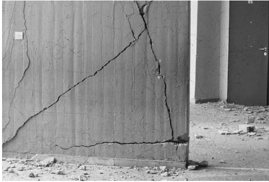
Figure 11.15 Shear wall failure: Kalamata, Greece (1986) failure to shear and simultaneously to bending.
