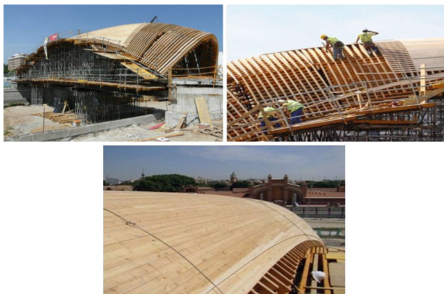
Fig. 2.30 Some details of the formwork
