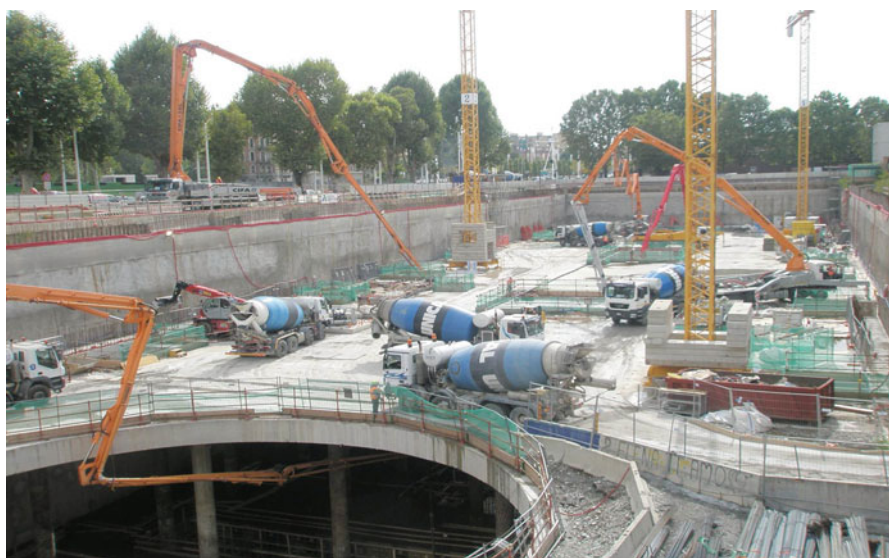
Fig. 2.9 Some views of the casting operation and equipment
