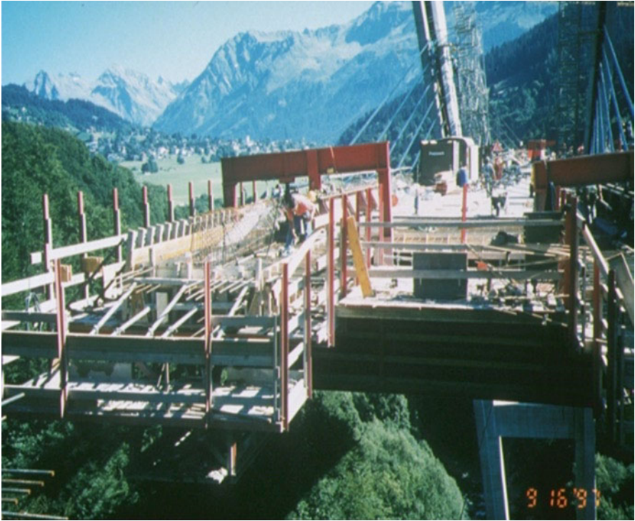
Fig. 21.9 Sunniberg bridge, form traveler
