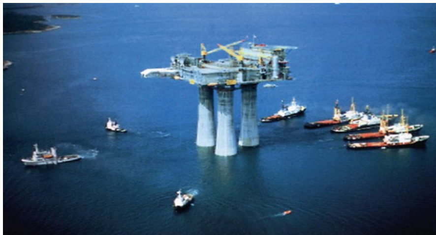
Fig. 20.1 Beryl A under tow to installation site, in 1975
