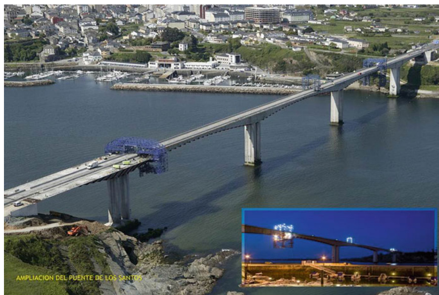
Fig. 2.18 View of the three platforms used on different parts of the bridge
