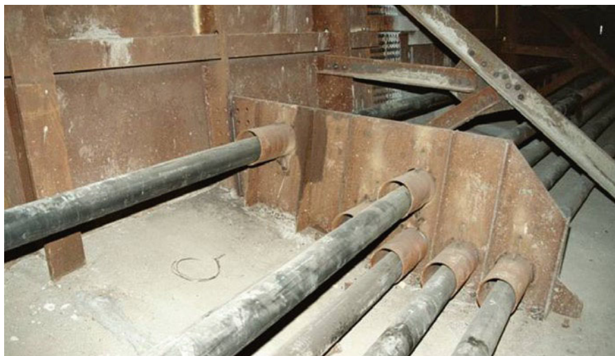
Fig. 23.13 External tendons' deviators
