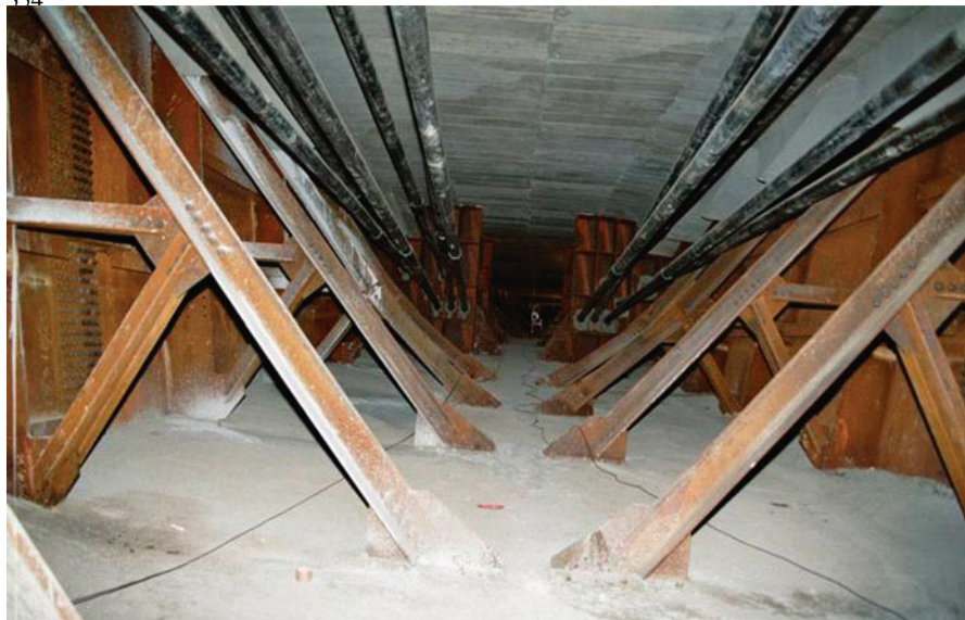
Fig. 23.12 Internal stiffeners
