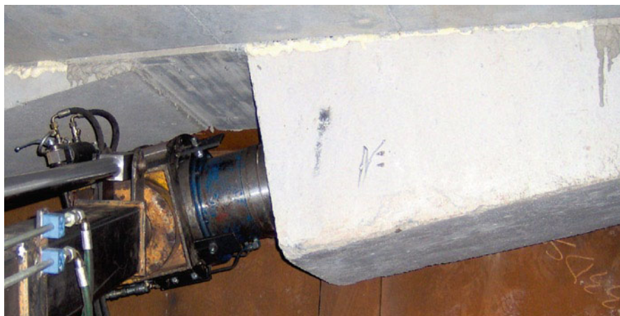
Fig. 23.8 Precast anchorage blisters
