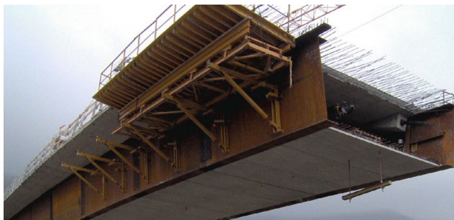
Fig. 23.7 Bottom and top flanges with formwork and scaffolding
