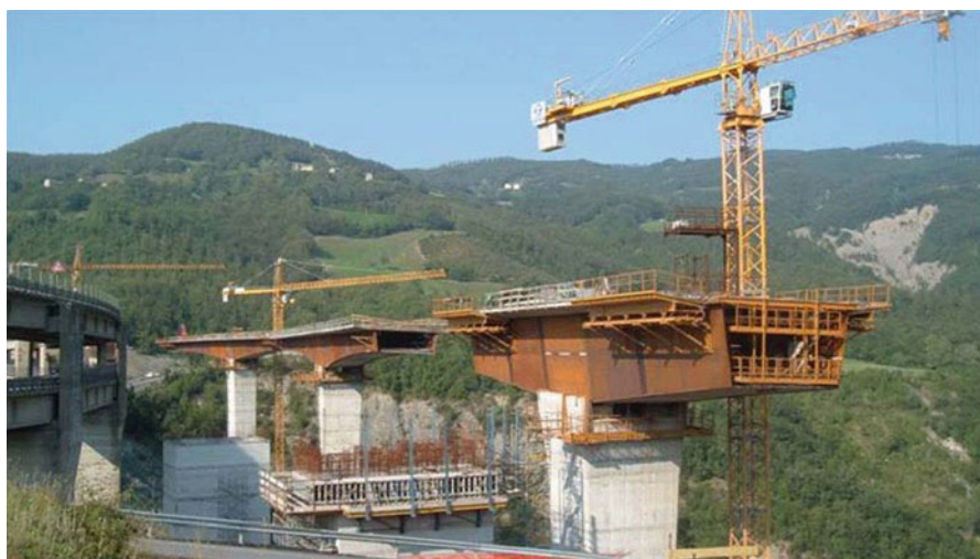
Fig. 23.9 Parallel construction of several hammers
