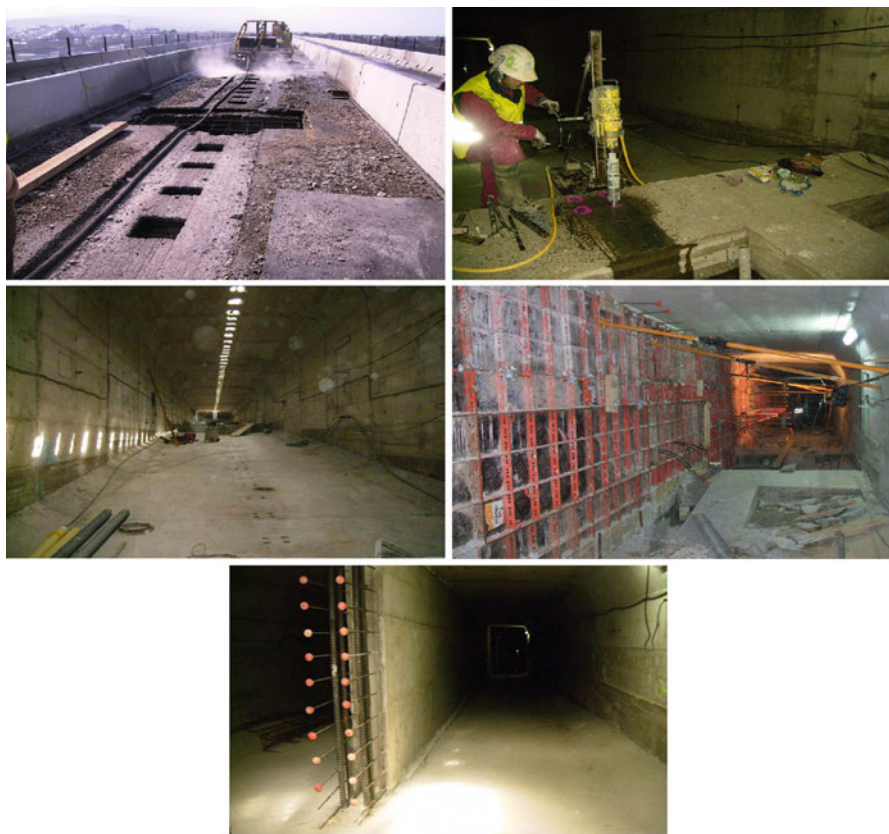
Fig. 2.16 Inner web with self-compacting concrete: drilling to place reinforcement at top slab , with hydrodemolition to avoid damage to existing reinforcement; in bottom slab , conventional drilling, accepting a certain percentage of affected bars; assembly of mild and prestressing steel
