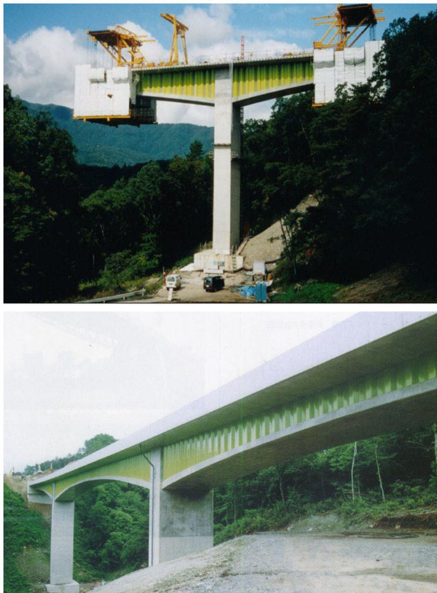
Fig. 22.18 Concrete bridge with corrugated steel web by balanced cantilever segmental construction
