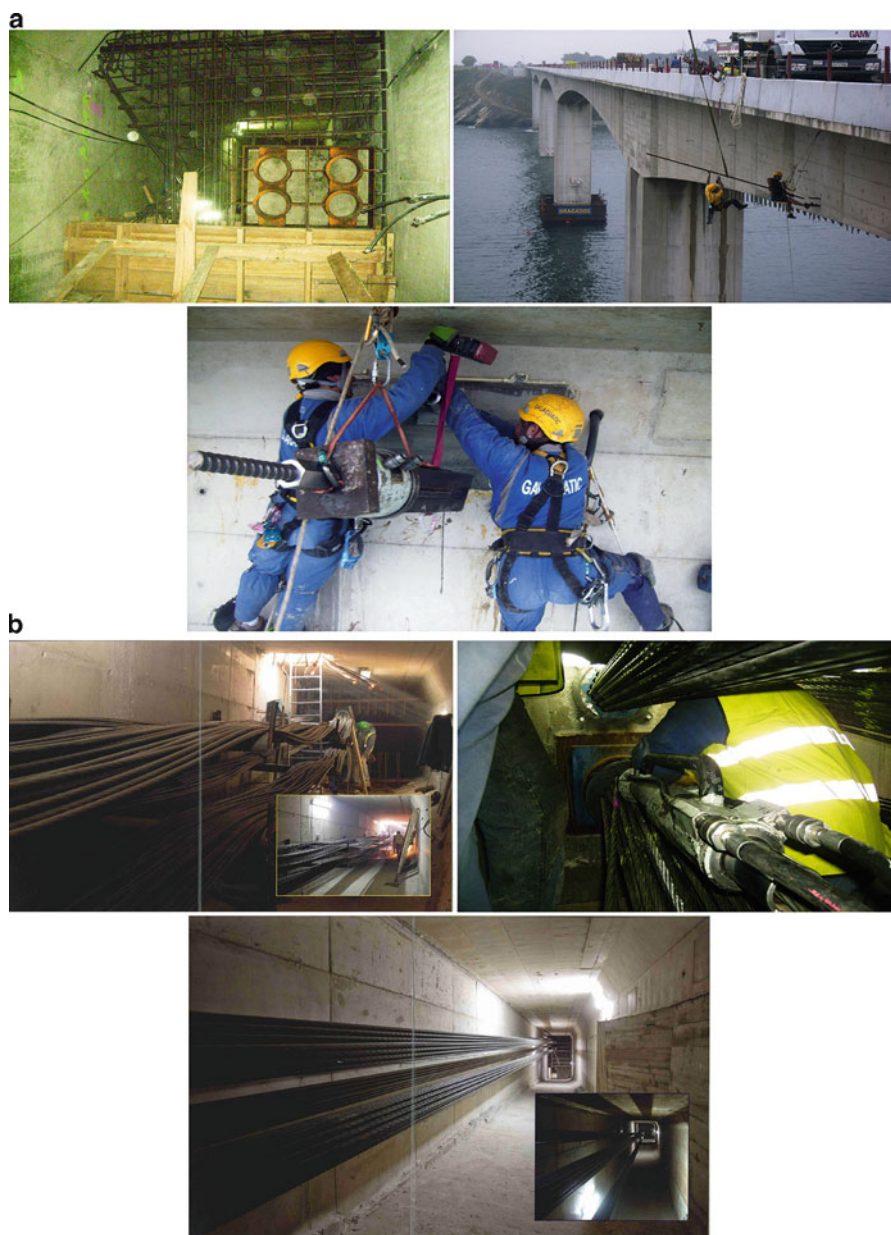
Fig. 2.17 Erection of inner web of self-compacting concrete. (a) Execution of deviators; Arrangement of connecting reinforcement to the existing box section. (b) Assembly of external prestressing
