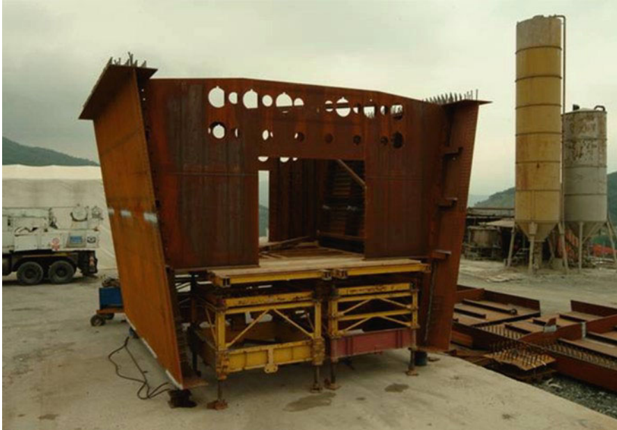
Fig. 23.5 Pier segment ready to be assembled
