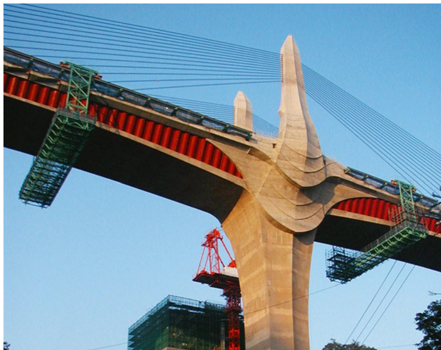
Fig. 21.16 Oumi-ohtori bridge, Frame joint
