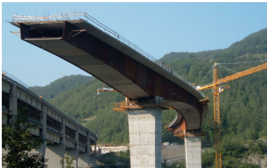
Fig. 23.10 Completed cantilever spanning 60 m
