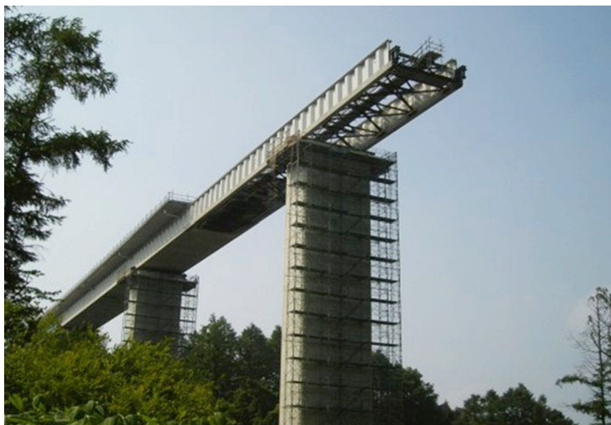
Fig. 21.12 Torisaki-gawa viaduct, launching (Courtesy of JH, Taisei)
