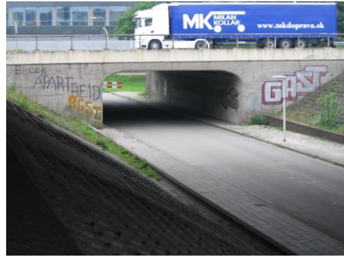
Fig. 8.3: Solid slab bridge deck
