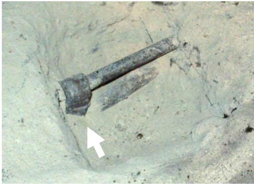
Fig. 1.2: Stirrup reinforcement in the form of a steel strip from 1905 at the Budapest University of Technology (opened during a reconstruction work, photo: courtesy of Tamás Lichter and Piroska Arany)
