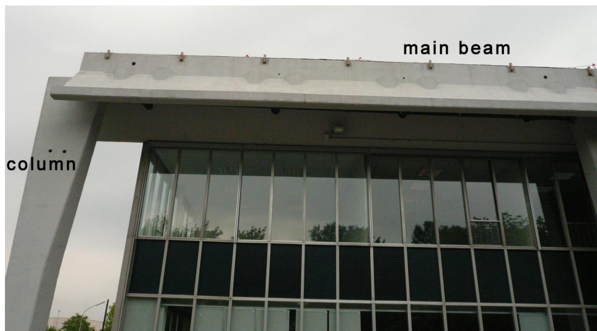
Fig. 11.1: View of a prefabricated roof with external and internal inverted-V main beams resting on tapered columns
