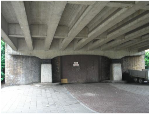
Fig. 8.2: T-beam bridge deck
