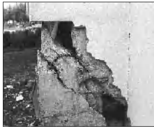
Figure 9.10. Failure of a short column
