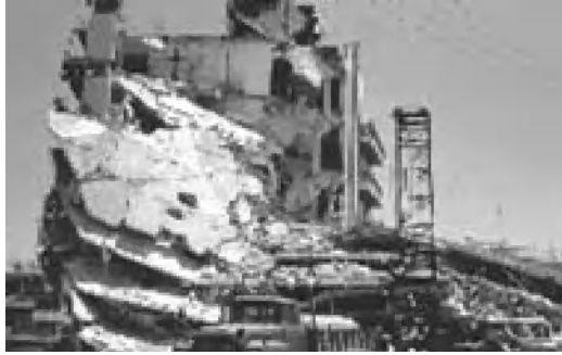
Figure 9.2. Collapse of a building showing overall torsion
