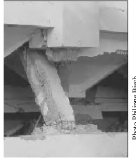
Figure 9.7. Rupture of a silo column with formation of a plastic hinge
