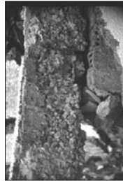
Figure 9.1. Poor-quality concrete in a column
