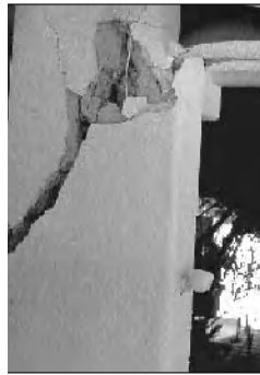
Figure 9.8. Rupture of a column showing the influence of the shear load
