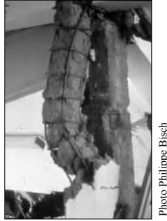
Figure 9.6. Rupture of a column due to buckling
