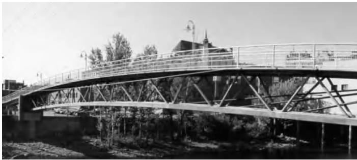
Figure 6.9. RPC pedestrian footbridge (Sherbrooke, Quebec, Canada)
