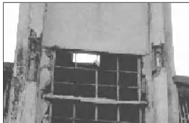
Figure 9.14. Rupture of the cover in a column due to a reinforcement tie bar
