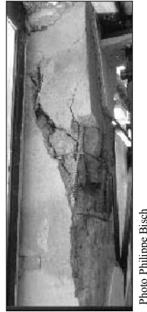
Figure 9.9. Failure of a column due to shear load
