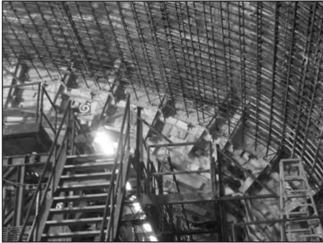
Figure 2.12 Wooden bulkhead against waterproofing in drill-and-blast tunnel
