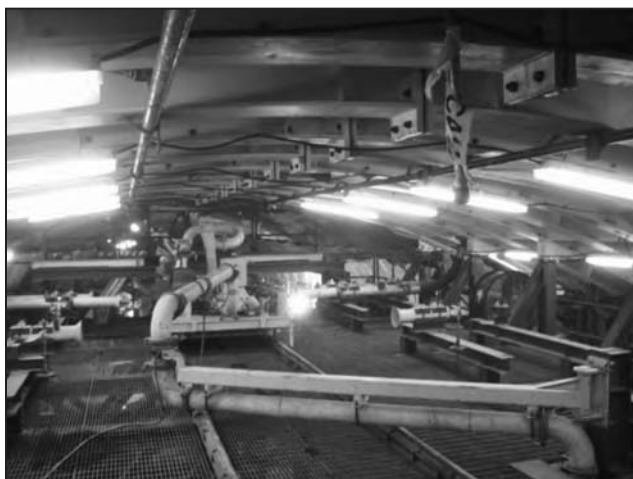
Figure 2.11 Standpipes to pump concrete through the formwork from a single location
