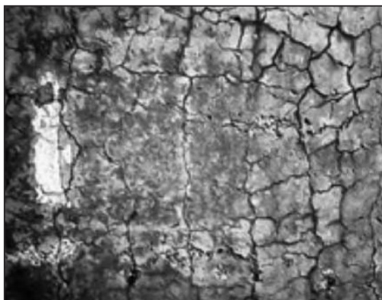
Figure 1.3 Examples of alkali-silica reaction between cement paste and reactive aggregates
