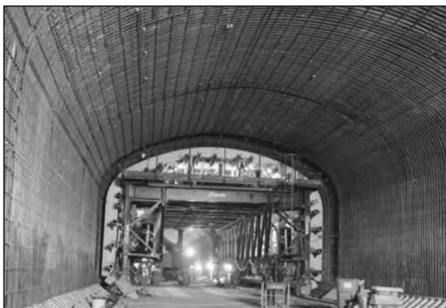
Figure 2.9 Tunnel concrete must be able to flow around reinforcement with limited use of immersion vibrators
