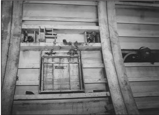
Figure 2.2 Typical steel form interior with window, with form vibrator at right and positioning spuds at top
