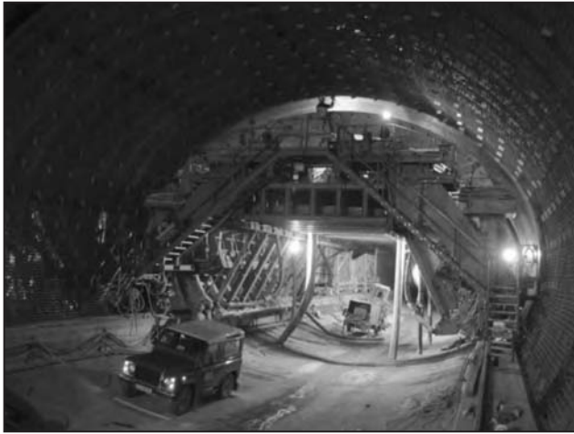
Figure 2.8 European-style form for NATM tunnel
