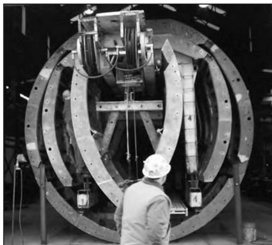
Figure 2.3 Telescopic formwork—collapsed arch and invert form on carrier inside expanded full round form
