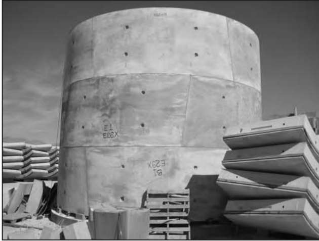
Figure 3.5 Trial rings to demonstrate good ring build
