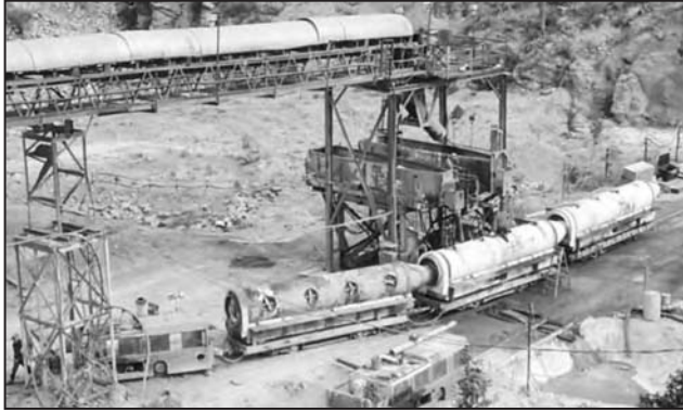
Figure 2.10 Moran cars waiting to be filled with concrete at the surface
