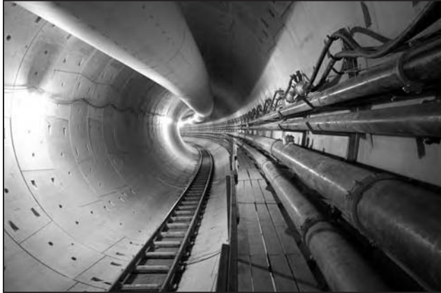
Figure 3.2 Completed SFRC segmental lining
