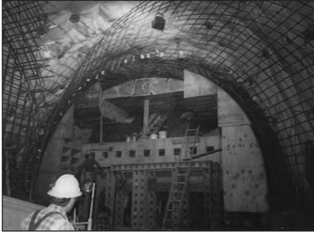
Figure 2.5 Modular wood forms shop-built for subway station
