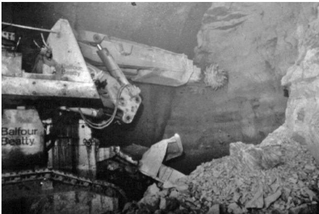
Figure 3.6 Excavation of an SCL tunnel using a roadheader.
