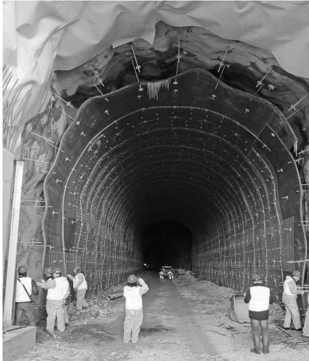
Figure 6.15 Drip-shed inside an SCL tunnel.
