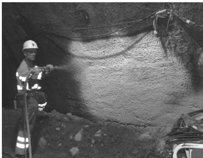
Figure 4.8 Spray-on membrane installation.
