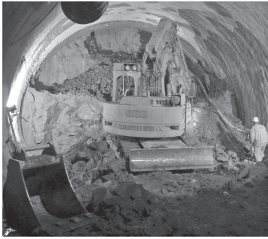
(a) Top heading, bench and invert
