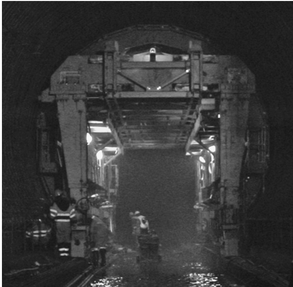
Figure 4.10 Formwork for cast concrete secondary lining.
