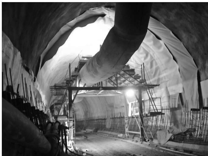
Figure 4.6 Sheet membrane installation.
