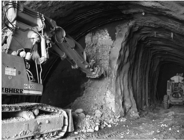
Figure 3.1 Excavation of an SCL tunnel in soft ground.
