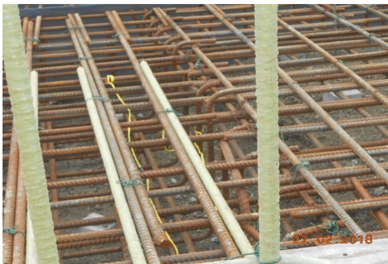
Fig. 11.3 Picture showing thermocouple with exposed wire sensors fastened to top and middle layers of rebar
