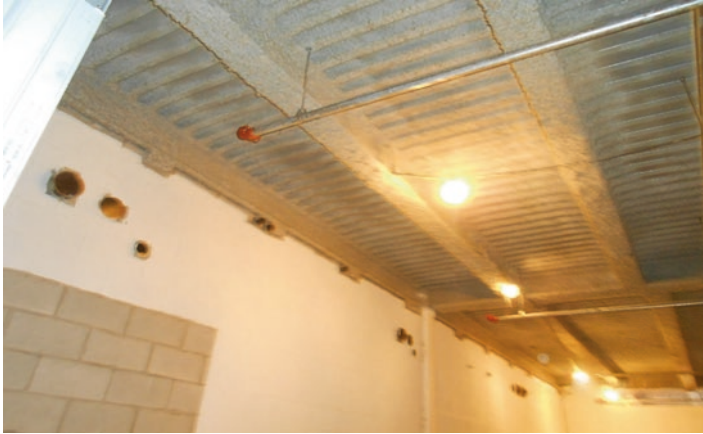
Fig. 8.14 Spray-applied cementitious material fireproofing
