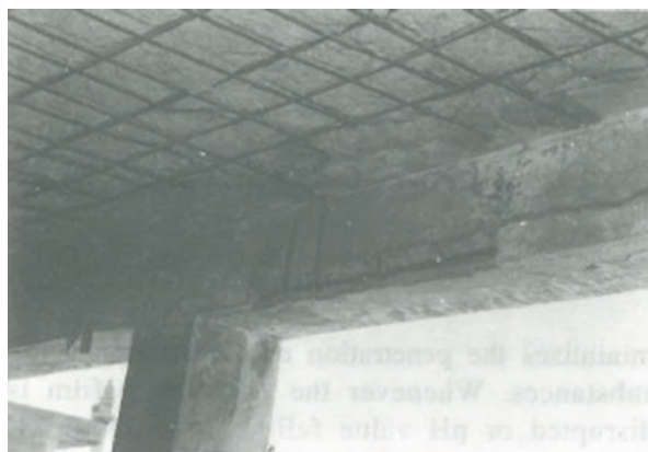
Fig. 10.2 The badly delaminated concrete soffit of a school corridor
