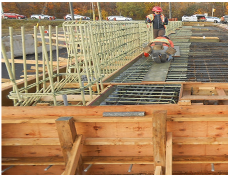
Fig. 10.6 GFRP and traditional rebar installation in progress
